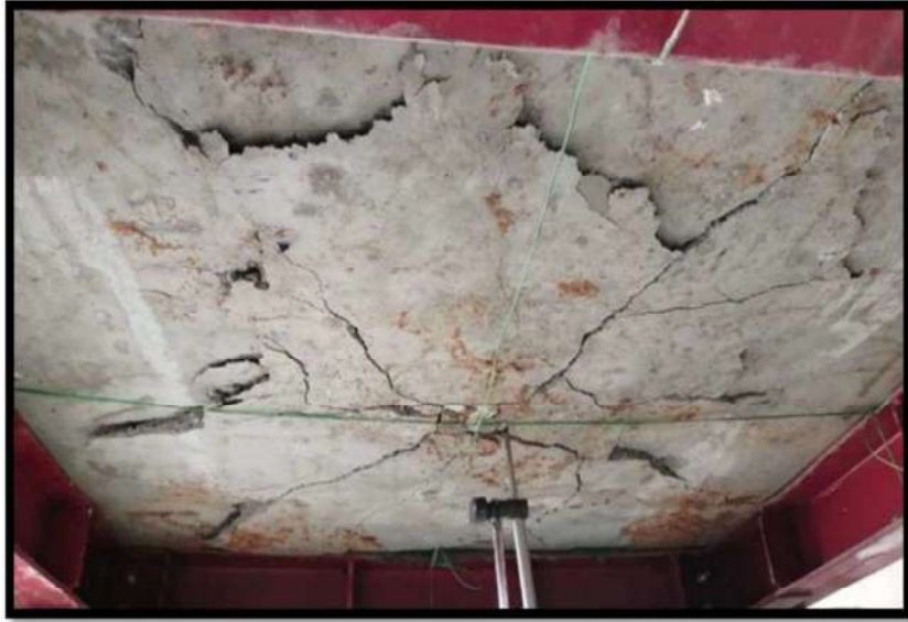
Figure 10: Failure mode of the specimen D150_S150
